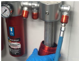
Unscrew lower section
